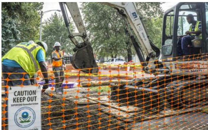
Soil cleanup of a Superfund site.
