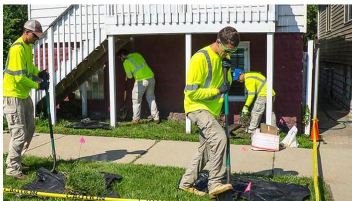
Soil cleanup on a residential property.
